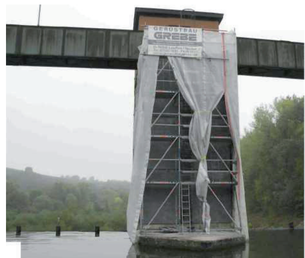
Fig. 12. Test repair of a pile of the Neckar weir at Horkheim
